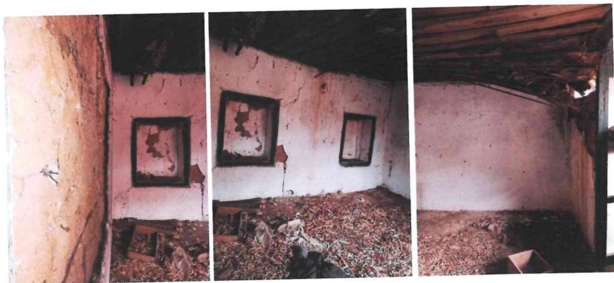
Figure 54. Ambient 8, majtas- suva me llac cemento
