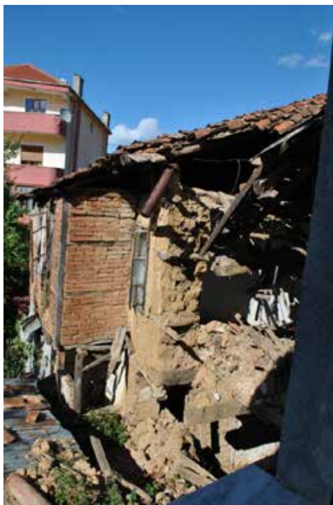
Three storey house in Pogradec built with mud brick walls
