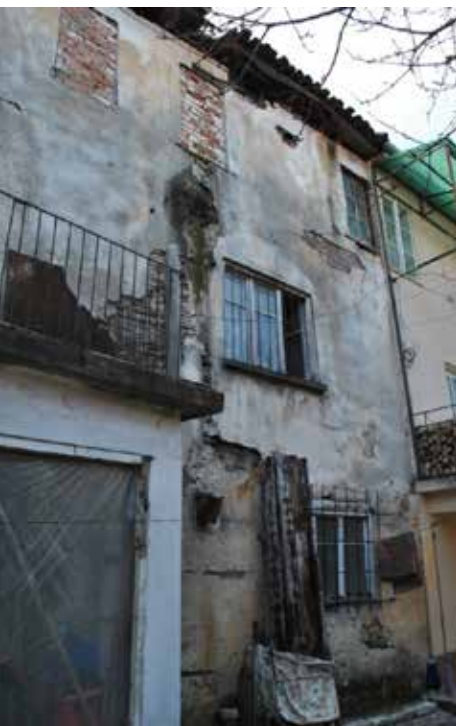
Three storey house in Pogradec built with mud brick walls
